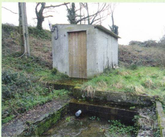
Station pompage Cosqueric.
